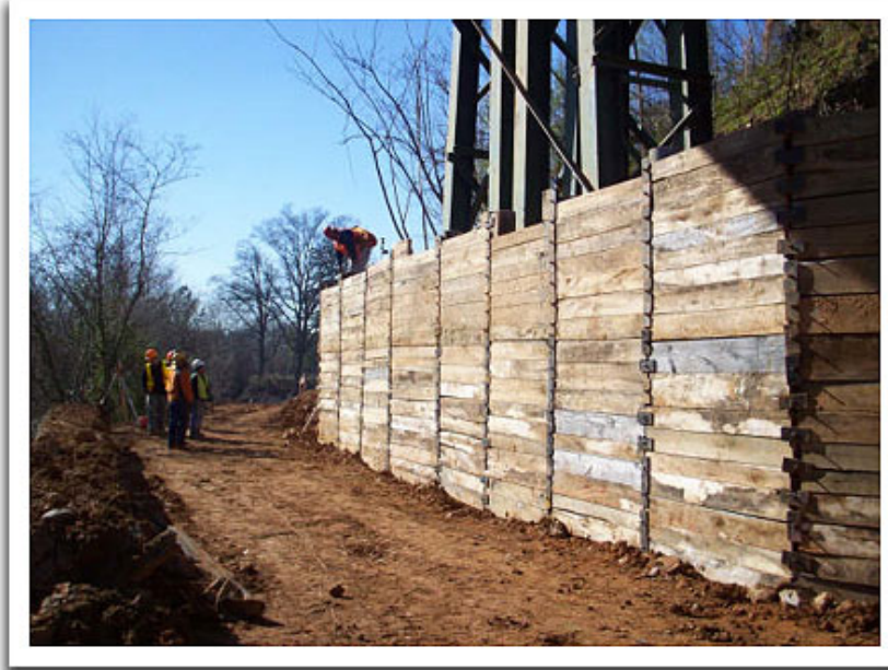
Little Sugar Creek Greenway– Charlotte, NC Pipe and Lagging Shoring Wall
